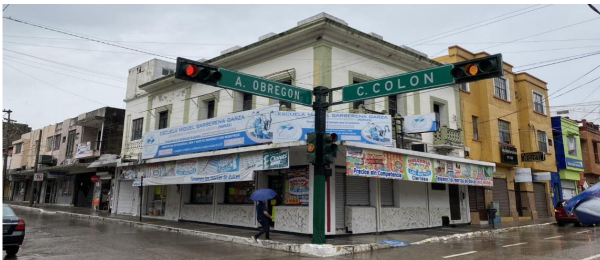
Figure 3. Use of existing lawn mowers in a building, where the 1st floor is used for a candy store for parties and the 2nd floor for a School
