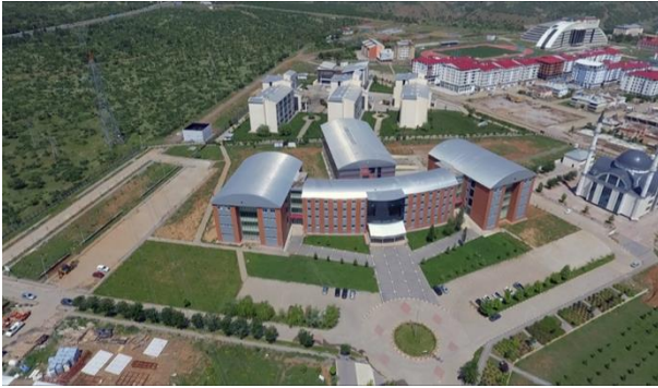
Figure 1. Overview of Bingöl University Faculty of Engineering and Architecture building (Available at: http://mmf.bingol.edu.tr/mansetler/muhendislik-mimarlik-fakultesi-1/ )
