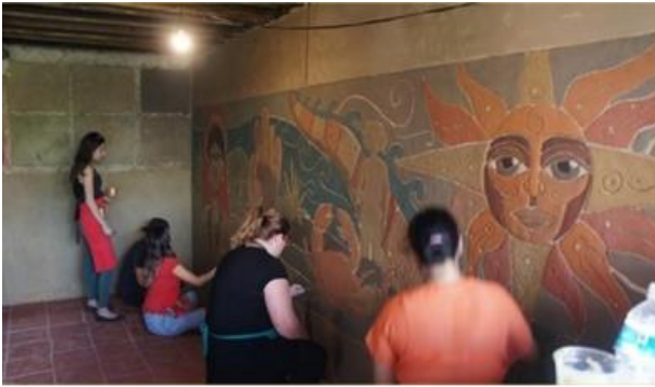
Figure 7. Finishing of the use of earth mortars in a wall
