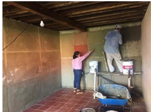
Figure 1. Image of earth test in walls
