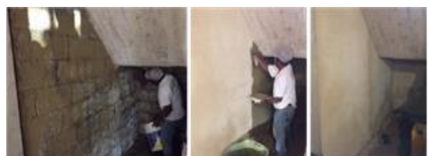
Figure 2. Image of earth mortar in walls surface
