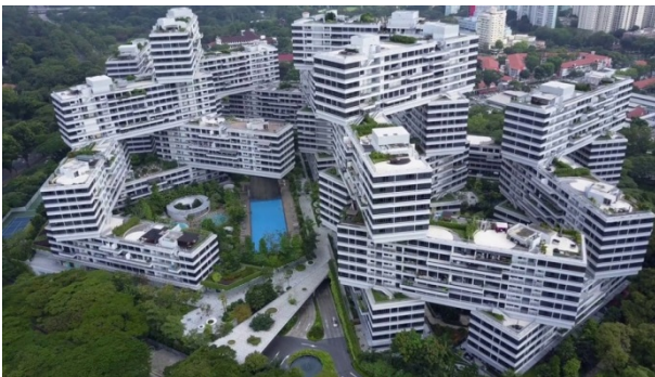
Figure 1. A perspective of the The Interlace residential project in Singapore [16]
