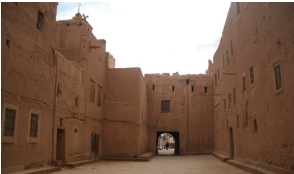
Figure 2. The raw earth construction in Tinejdad oasis
