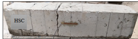
Figure 16. Crack patterns of prism for control specimen after loading
