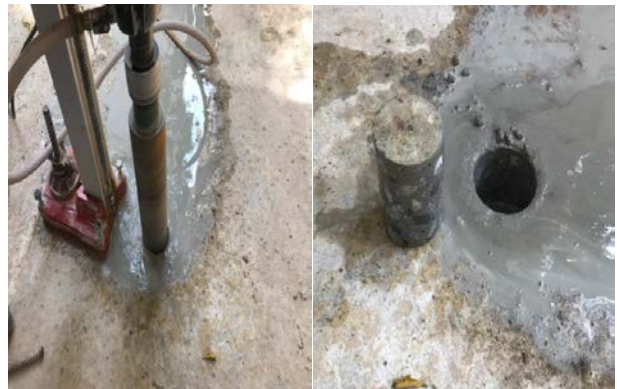
Figure 41. Core Cutting Apparatus' and Core Extraction at Site
