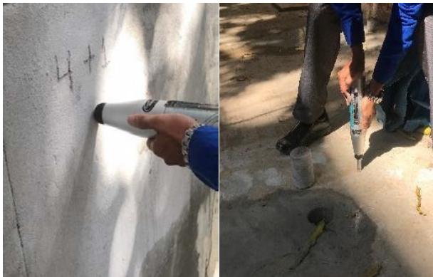
Figure 39. Rebound Hammer Test at Site
