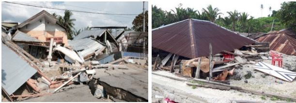
Figure 6. Building damage due to earthquake in Halsel, 2019
