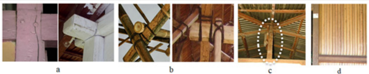
Figure 12. Building construction: (a) Button System (b) Bond system, (c) Tiang raja (king pillar), (d) gaba-gaba (sago stem), (Source: author)
