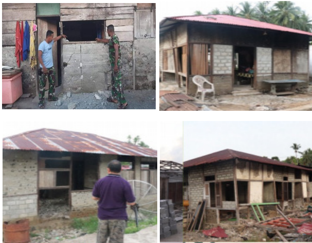
Figure 7. Falakanci house that survived the 7.7 mag earthquake in Halsel, 2019
