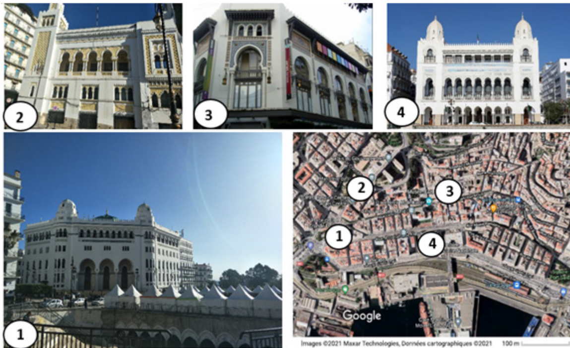
Figure 3. Locations of neo-Moorish buildings in Algiers (Source; Photos (1, 2): Authors, 2019, Photo (3): https://www.tripadvisor.fr/ Photo (4): https://www.inter-lignes.com/la-wilaya-dalger-autorise-la-reprise-de-certaines-activites-professionnelles/ ,
