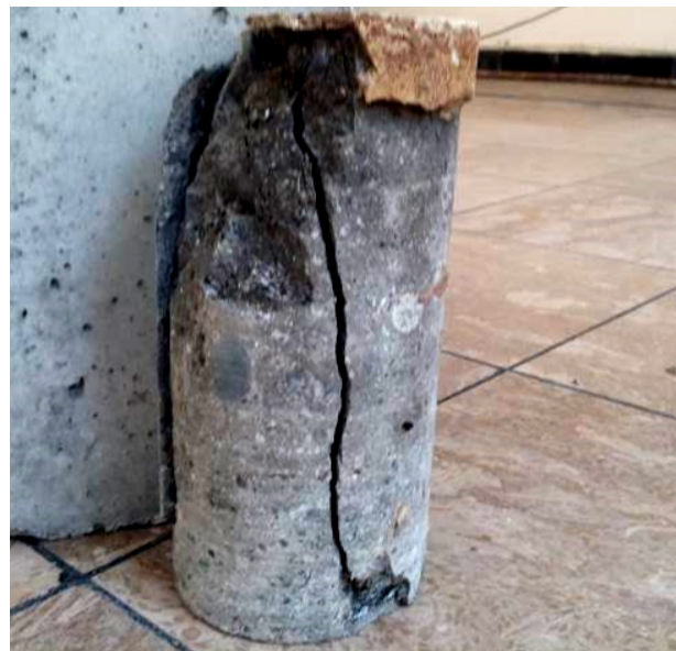
Figure 5. Failure form of plain shotcrete specimens
