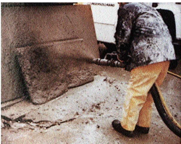
Figure 4. Panels sprayed with Shotcrete
