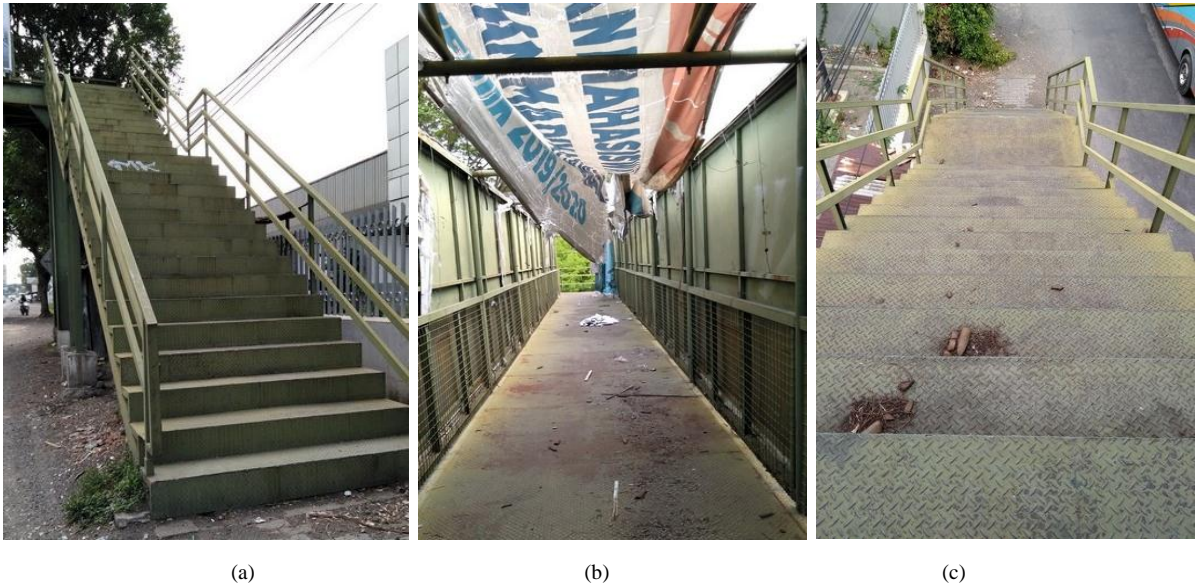
(a) height of footbridge steps (b) footbridge walking path (c) footbridge steps viewed from upstairs
