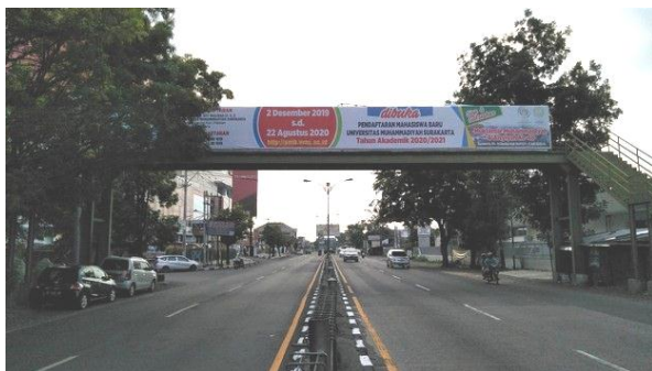
Figure 3. Pedestrian footbridge viewed from U.M.S. Campus direction
