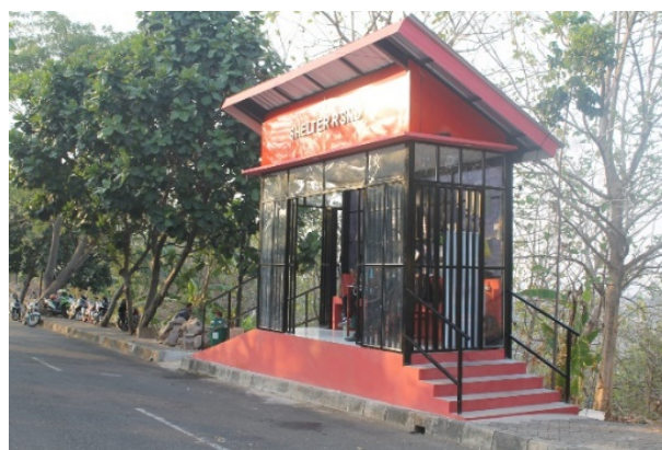
Figure 1. The common shelter condition in Undip
