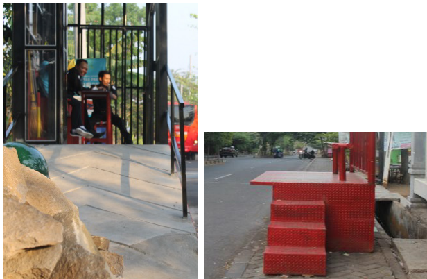
Figure 4. Condition of ramp, stairs, and furniture
