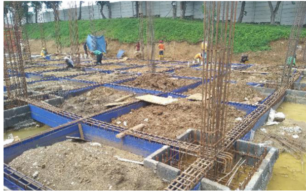
Figure 1. Shop-House Project using woven polyethylene formwork
