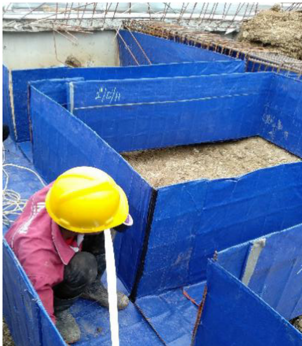
Figure 2. Road Pavement Project using woven polyethylene formwork
