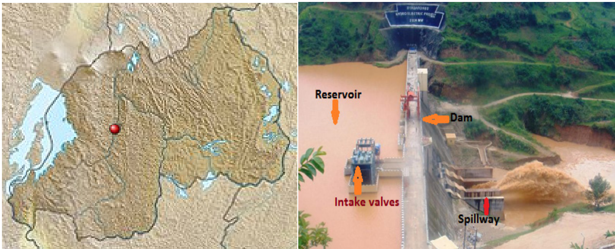
Figure 4. Location of the Nyabarongo I Hydropower plant and Dam [3]
