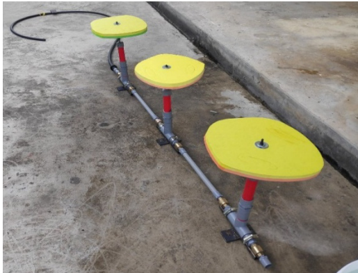
Figure 7b. Pumps connected in series
