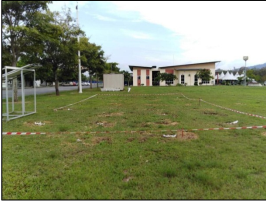
Figure 2. Grounding system installation site
