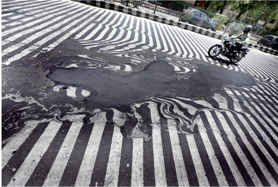
Figure 3. Air and especially surface temperatures are higher in the central city than surrounding suburban and rural areas. This melted asphalt is in an Indian city, where pedestrians crossing the street have been known to lose their shoes to the melted, sticky road surface. (Photo by Harish Tyagi/Epa/REX/Shutterstock (7978897g))
