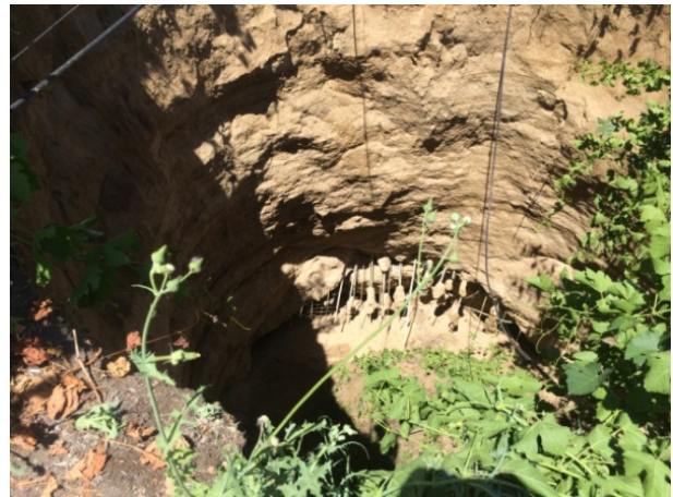
Figure 2b. Looking down into the tunnel; vine vegetation and wires from trellises on the surface fell into the opening.
