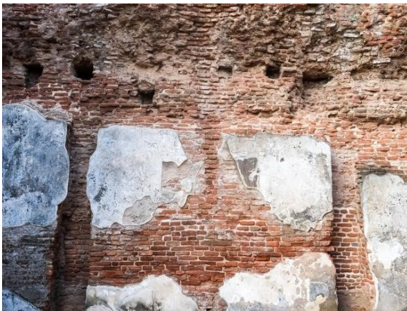
Figure 1.4. Existing plastering on the walls of the palace
