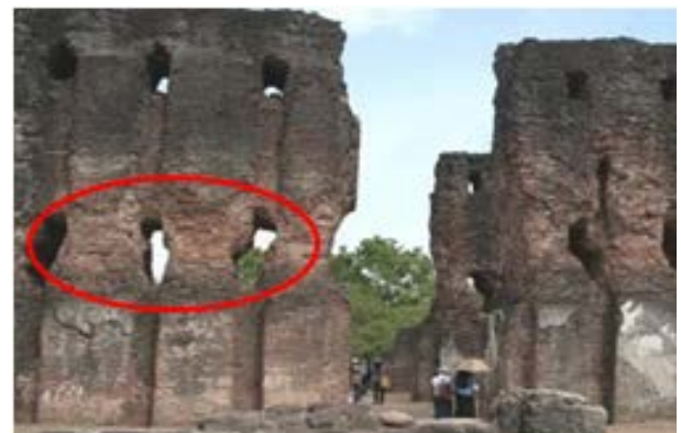
Figure 1.2. It is assumed that large beams had been fitted to these huge grooves
