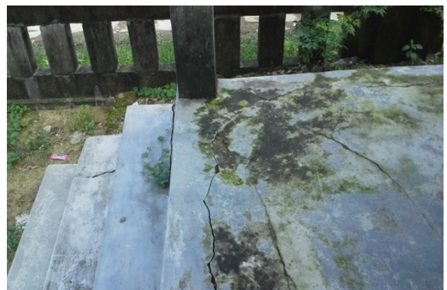
Figure 5. Local resident's house with poor concrete slab at entrance
