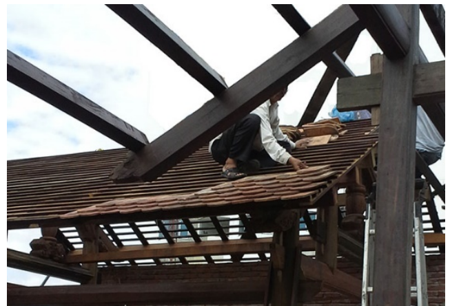
Figure 10. Installation of roofing tile at a new residential construction
