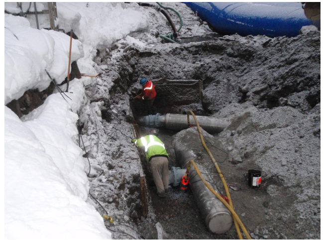
Figure 6. Infiltration gallery prior to covering with 916 mm, minus rock and coarse rock 25 – 50 mm
