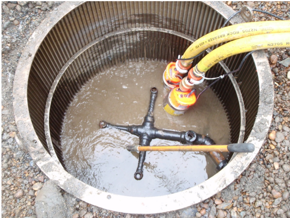
Figure 2. 1219 mm (48-in) well with jetting nozzles
