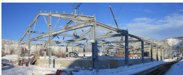
Figure 3. Dawson City wastewater treatment facility during construction in February, 2012
