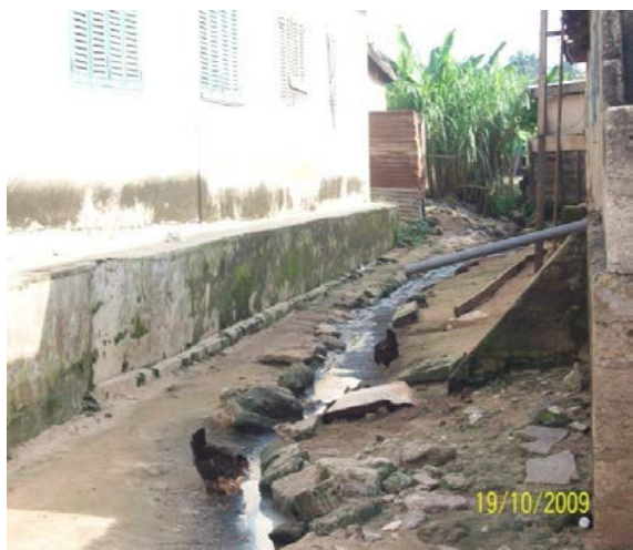
Plate 10. Poor drainage between
