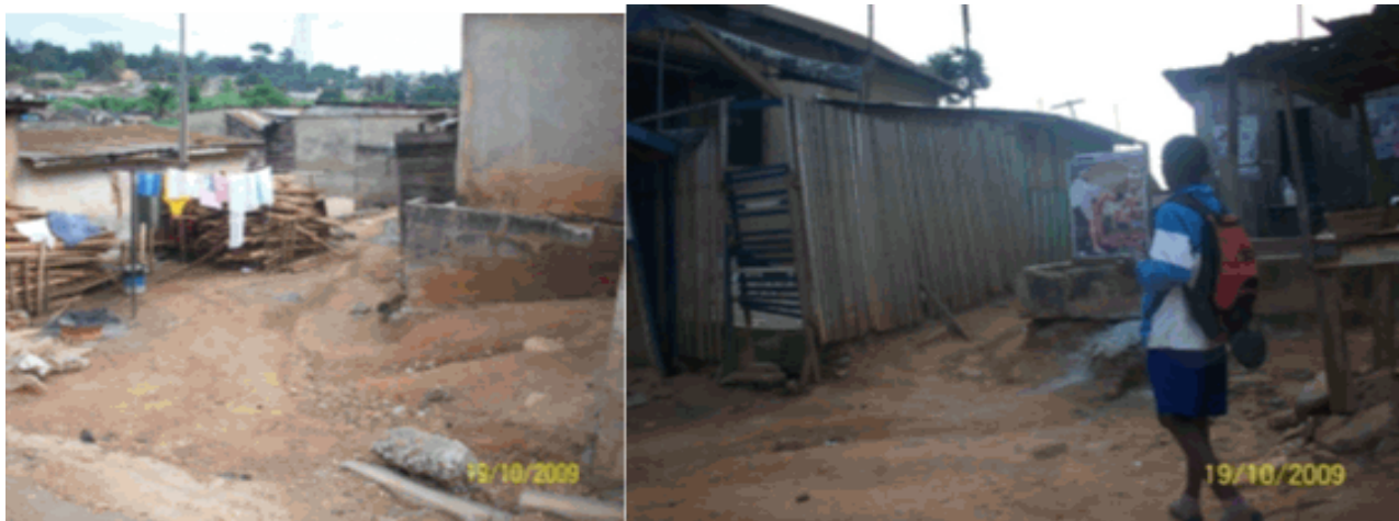
Plate 2. and Plate 3. Poor Access routes in Anloga -Sobolo
