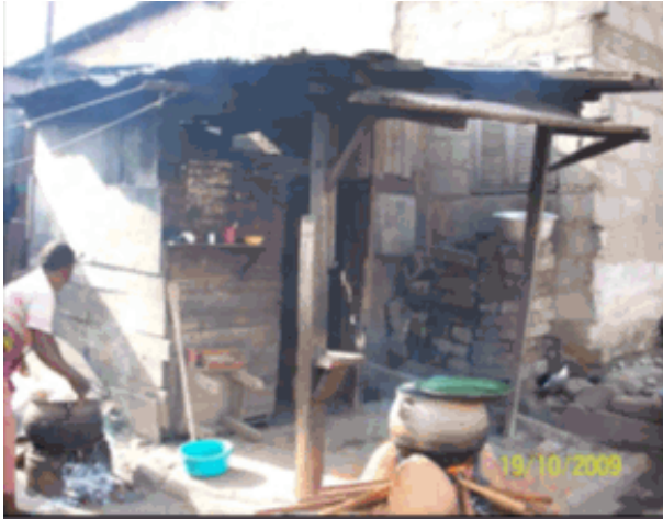
Plate 6. unfinished home with wooden building extension
