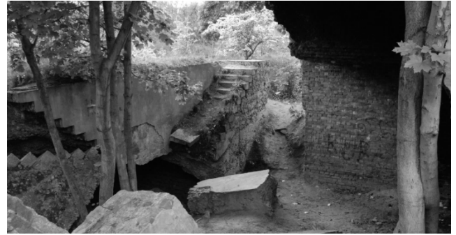
Photograph 1. Fort IV in Poznań (author: A. Sinięcki).
