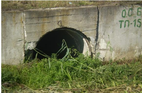
Figure 4. Degradation of the material between the terminal and these align tube RTP-100
