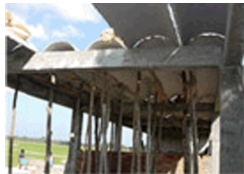
Figure 23. The ferro-cement jack arch shells roofs for classrooms (DesignShare: Designing for the future of learning 2013)
