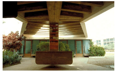
Figure 6. The triangle canopy works as a courtyard between the classrooms (Aga Khan Trust for Culture 1979)
