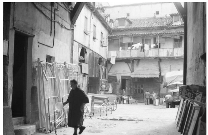
Figure 1. 'Corrala' typical Madrid dwelling: (16 th Century) 18 m x 32 m dwellings around a central patio
